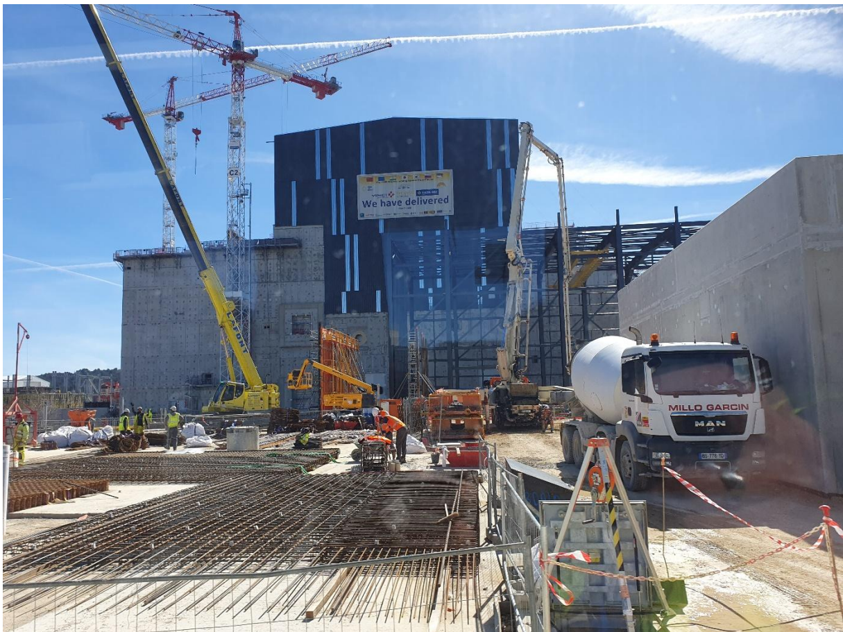
Figure 1: The assembly hall in the ITER construction site (source: author)
