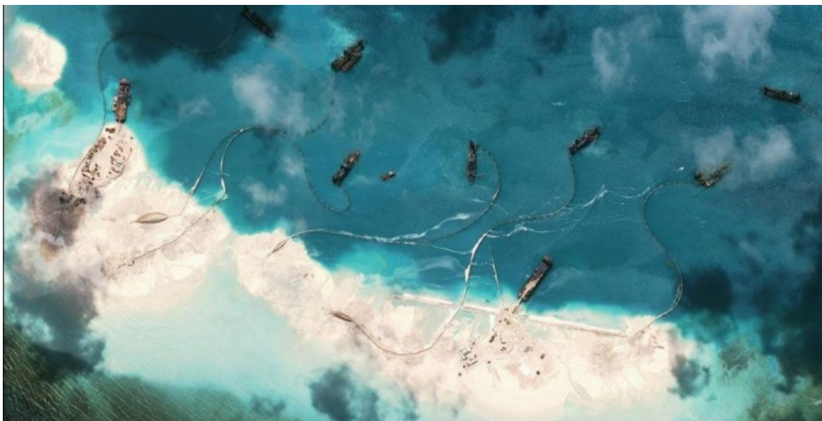
Figure 6: Chinese dredging activities at Mischief Reef on 16 March 2015
