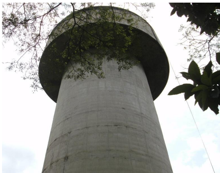
Fig.21: The Ughelli North Urban Water Board Division tower
