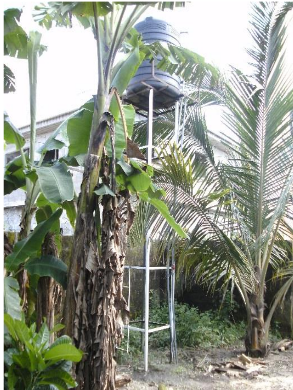
Fig.10: This is the way a private water tank looks like.
