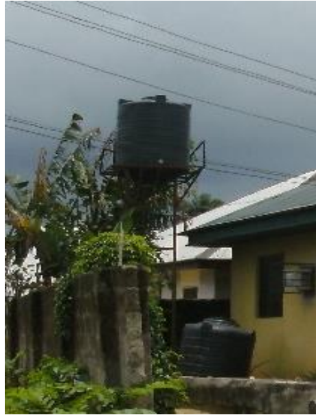
Fig.11: The picture shows that the cesspit and the tank are too close.
