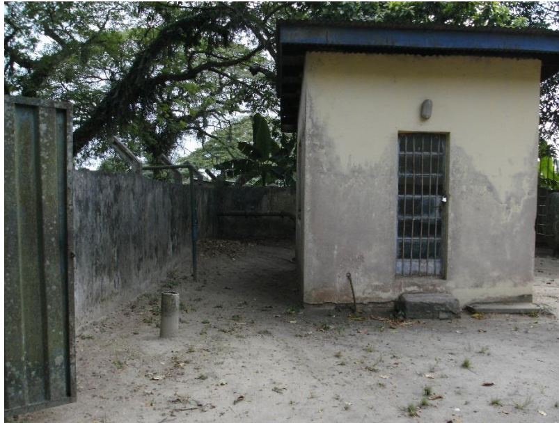
Fig.24: The equipment house in the compound of Ughelli North Urban Water Board Division.
