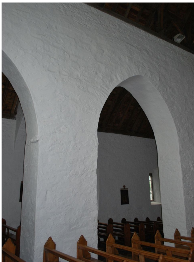
Fig. 96: Holycross Abbey, twelfth-century north arcade of the nave.
