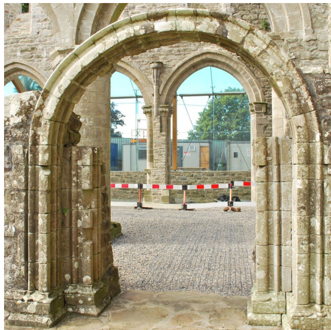
Fig. 43: Boyle Abbey, processional doorway in the north east of the cloister/east end of the south aisle.
