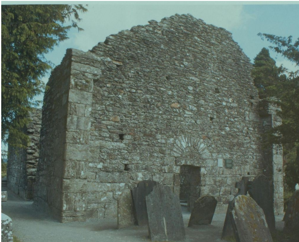
Fig. 17: Glenadlough, the Cathedral from the west.
