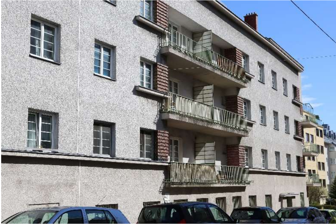
Abb. 114: Schmid/Aichinger, Somogyihof , 1927-1929, Fassade Gusenleithnergasse.
