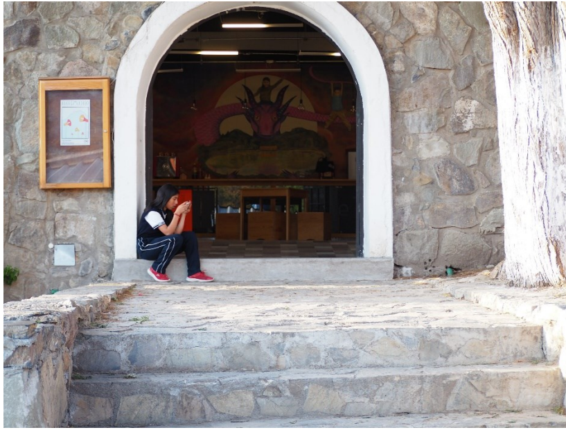
Figure 4. Cine Too entrance. Photo: Rodrigo Ruiz. 2019
