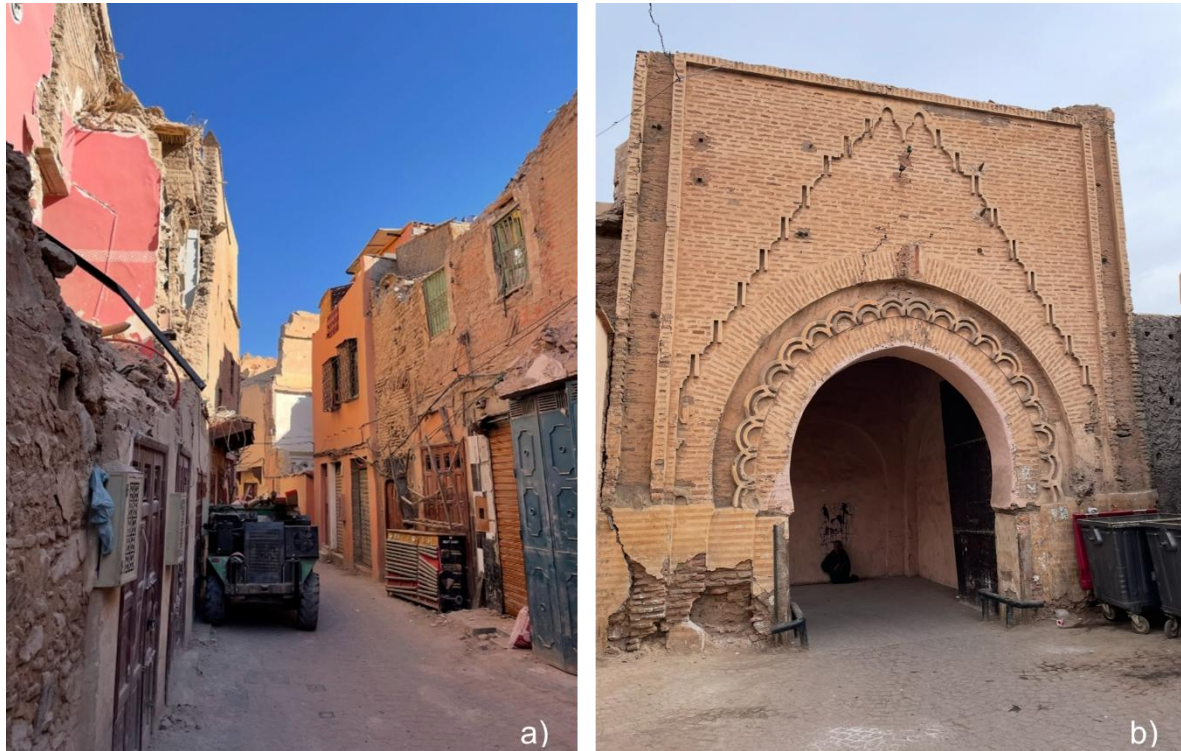
Fig. 7: a) Earthquake damages in the tannery quarter (Photo: V. Immervoll, Marrakech, September 2023); b) Earthquake damages on Bāb Dbbāgh (Photo: V. Immervoll, Marrakech, February 2024)
