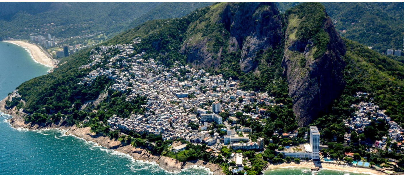
Figure 02. Vidigal slum, an urban informal settlement located in one of the most valued areas of the city of Rio de Janeiro, Brazil.
