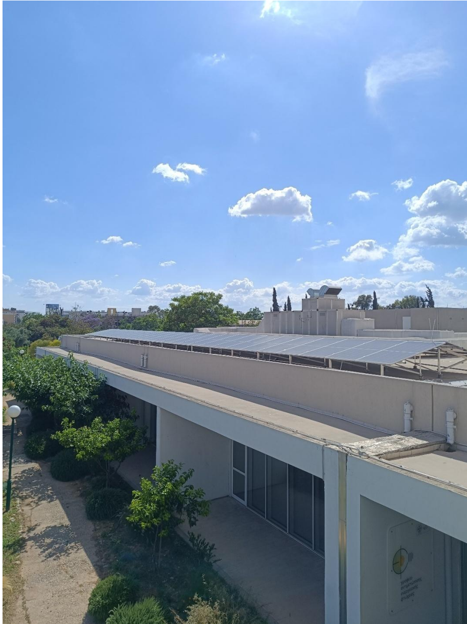
Photo 1. The solar panels over GAEF (Photograph by Ektoras Leventis)
