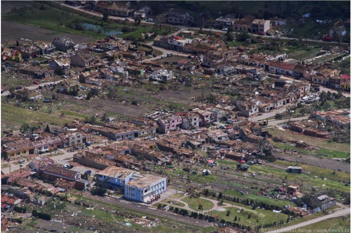
Abbildung 2: Schadensbild der 2021 Tornados in Tschechien. Quelle: Damage Survey of the Violent Tornado in Southeast Czechia on 24 June 2021 (Púčik, et al., 2024).
