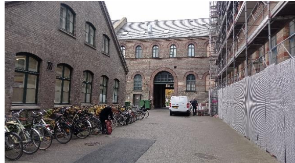
Figure 17: Yard 6, view towards building 12, building 20 on the left. Source: Author. .
