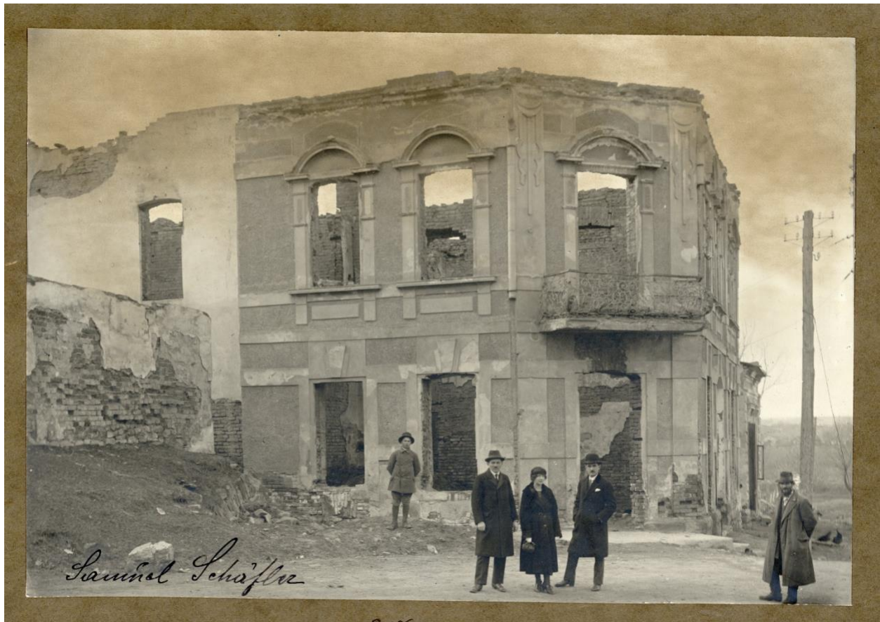
Figure 35. Building in Wijnitz destroyed by fighting on the front during World War I. Source: JDC Photo Collection NY_04539
