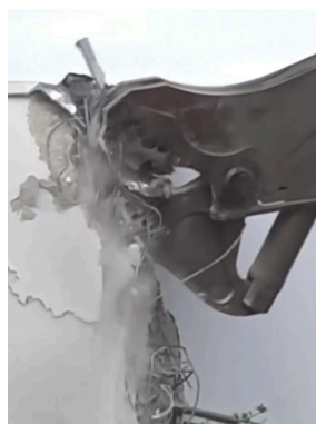
Figure 3 Demolition crews are tearing down the classroom building at Marjory Stoneman Douglas High School, where a mass shooting happened (@foxnews, 2024).
