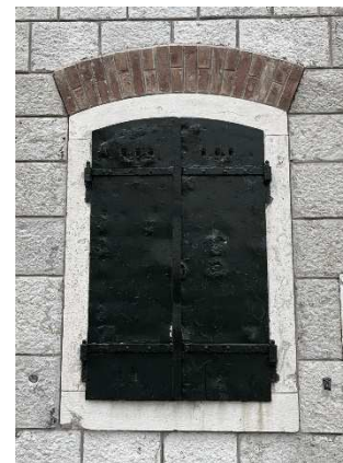
Abb. 7: Lager in Gruž, Dubrovnik, Fenster, Detail.
