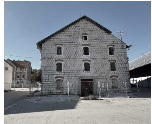
Abb. 6: Lager I (Nord), Sinj, Ostfassade.
