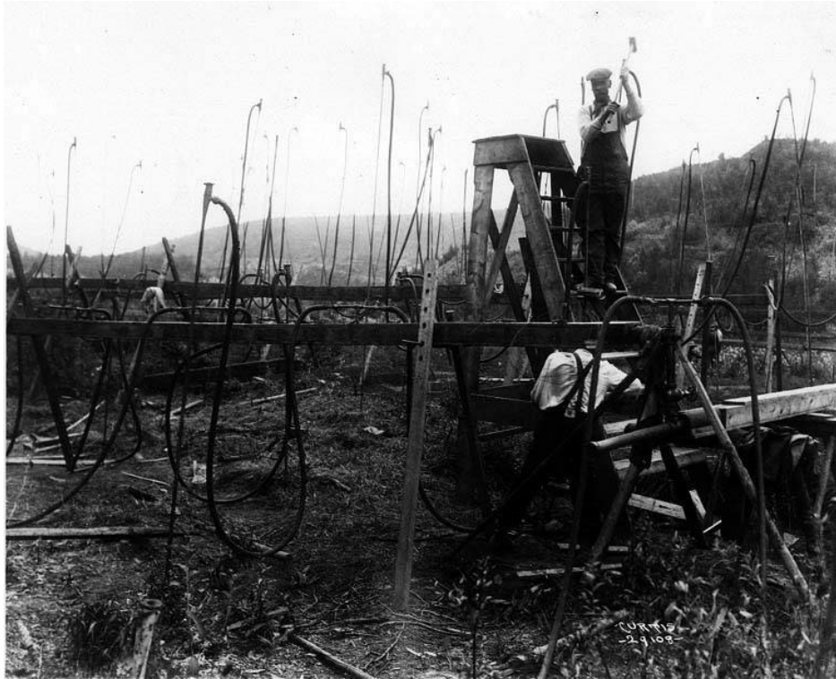
Figure 19: Driving steam pipes into the frozen tundra to thaw it, preparatory to dredging for gold, 1914; Photograph: CUR1134, Asahel Curtis Collection, Special Collections, University of Washington Libraries. Courtesy of the University of Washington Libraries.
