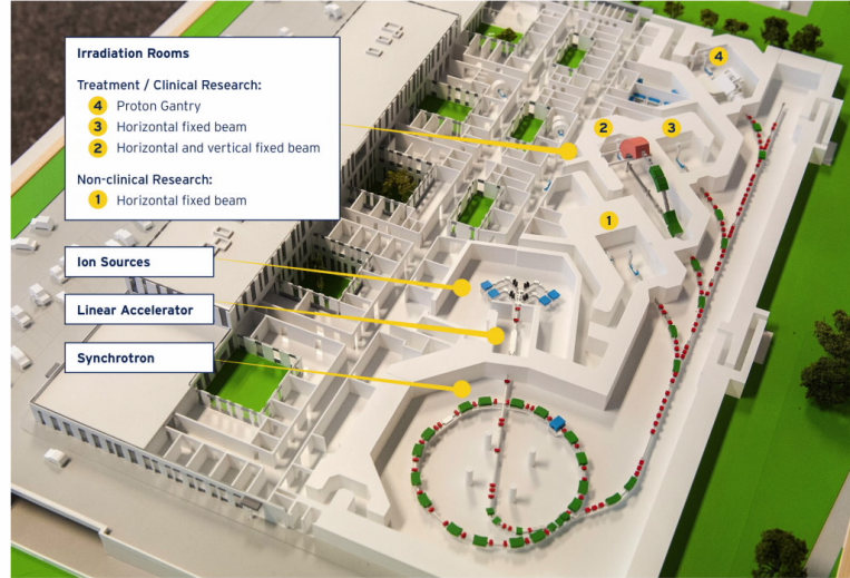
Figure 1.1.: Overview of the MedAustron facility, used with permission from MedAustron [10].
