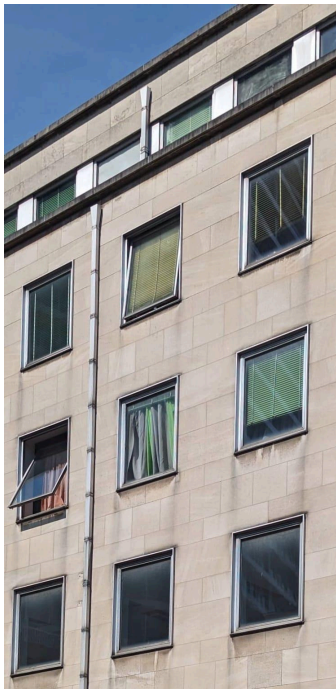
Figure 7. Windows at façade Rue Defacq. Photo by the author, 2024.
