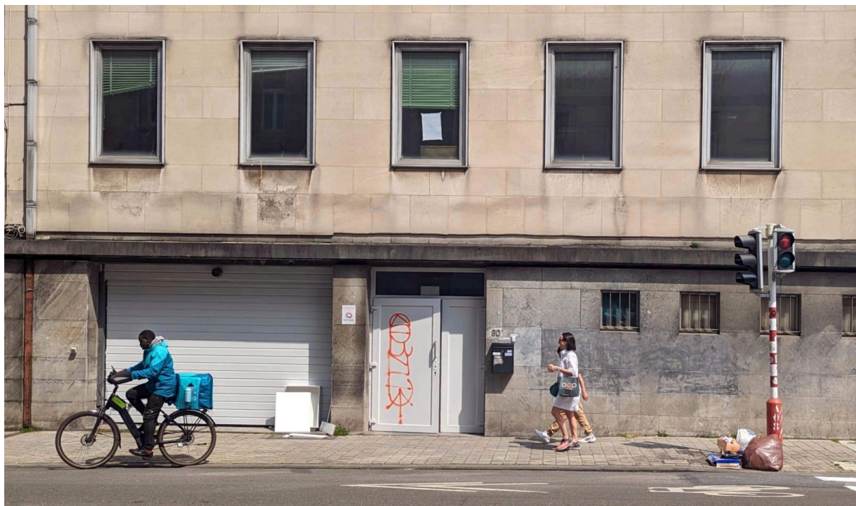
Figure 6. Façade of the entrance used by the occupants at Rue de Livourne. Photo by the author, 2024.
