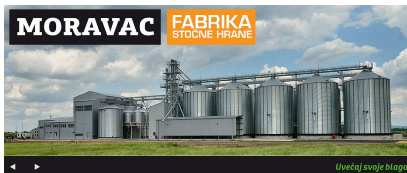
Figure 34: Production Plant of Moravac livestock Feed in Krnjevo
