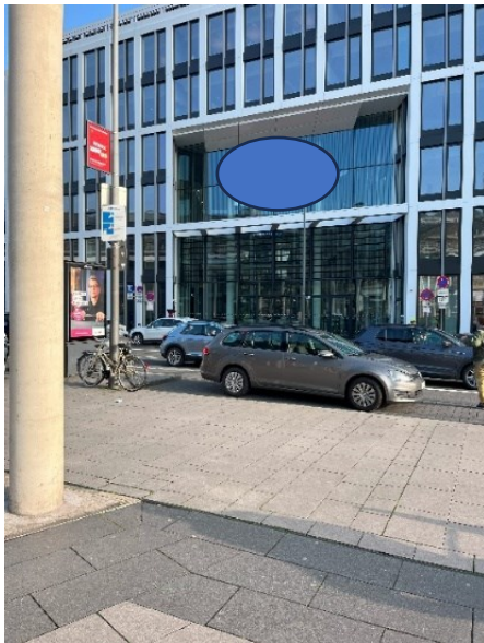
Photo 1: The front of the building
