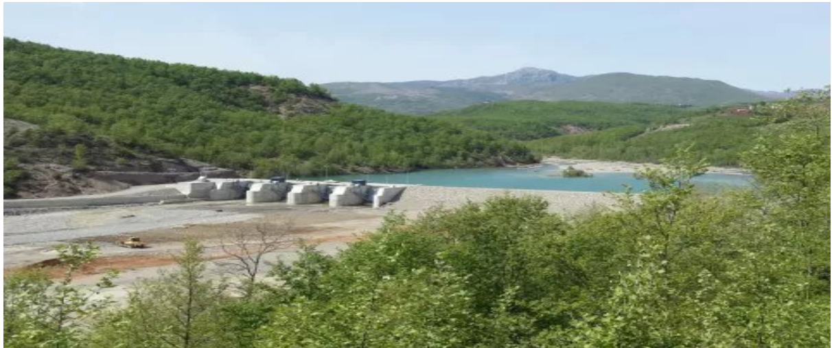
Picture 1 – Rapuni Hydropower Plant- Photo from Reporter.al, 2016
