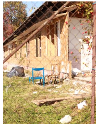
Figure 2.20: A "bostel" before demolition, 14 October 2018
