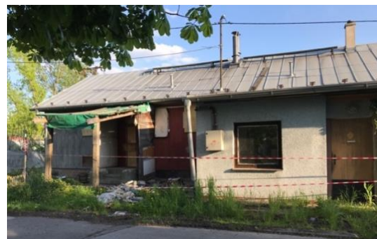
Figure 2.21: Vacant house, 8 May 2018
