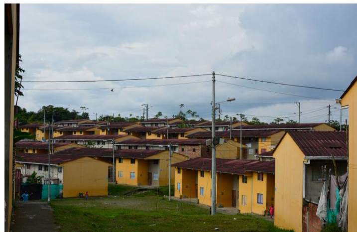
Figure 9: View of the planned San Antonio housing project. Retrieve from: Buenaventuraenlinea (08.2018) https://buenaventuraenlinea.com/proyecto-todos-san-antonio-se-busca-fortalecer-tejido-social-comunitario-buenaventura/
