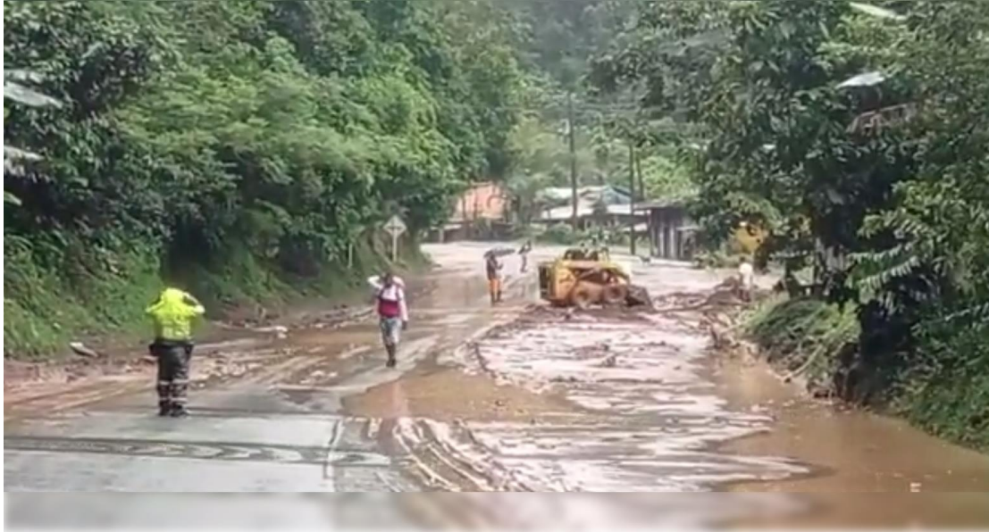
Figure 11: San Juan River flooding in Buenaventura. Q'hubo Cali (2022). Retrieve from: https://www.qhubocali.com/asi-paso/via-a-buenaventura-cerrada-por-desbordamiento-del-rio-dagua/
