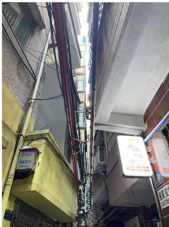
Figure 22 Wires and tunnels between buildings in Shipai village. Photo by author.
