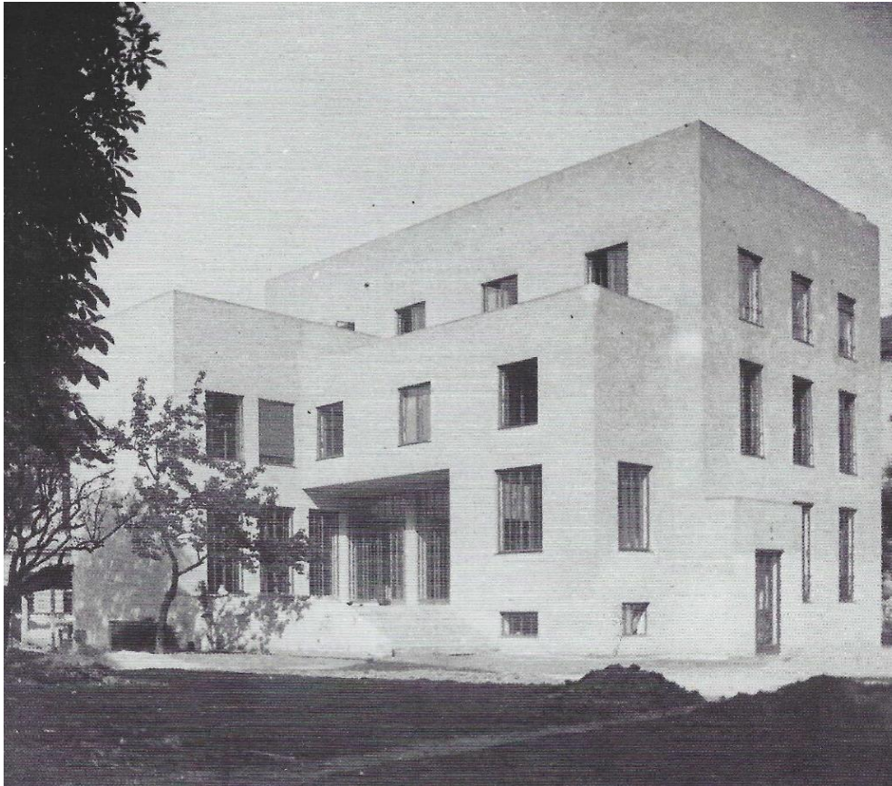
Abb.: 13 Haus Wittgenstein-Stonborough, Paul Engemann/Ludwig Wittgenstein 1926-1928 Bildquelle: Paul Wijdeveld, Ludwig Wittgenstein.Architect, Cambridge, Mass. 1993, S.15.
