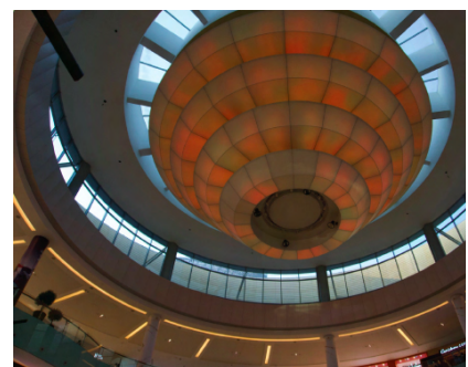
Figure 47 Dome, Dubai Mall (Riedl, 2022)
