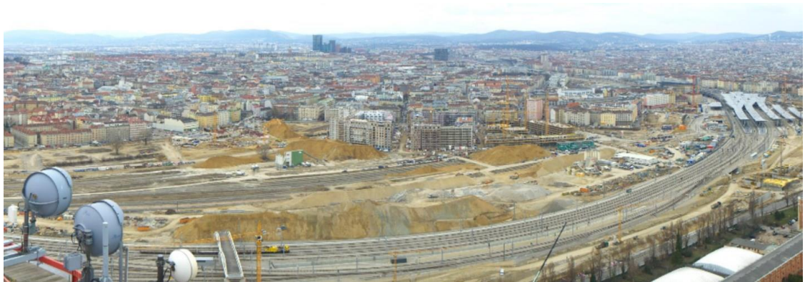
Aerial image of Sonnwendviertel construction. Source: Seidl, 2013. Accessed: June 6, 2021. Sent via temporary we-transfer link.
