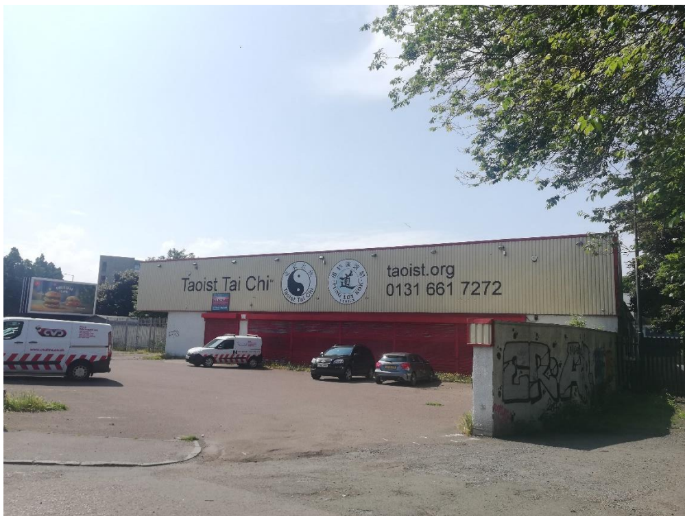
Former industrial unit to be redeveloped into housing. Source: Author
