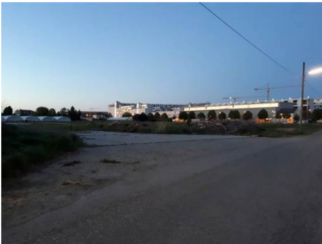
Figure A2: Location 1 seen from a distance when standing on the street “An der Schanze”.
