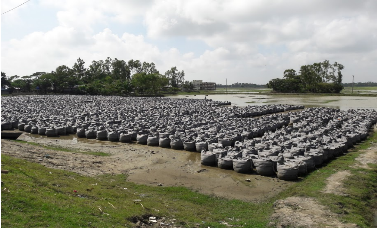
Figure: Geo-Textile bags for reduce River bank erosion in the Study area
