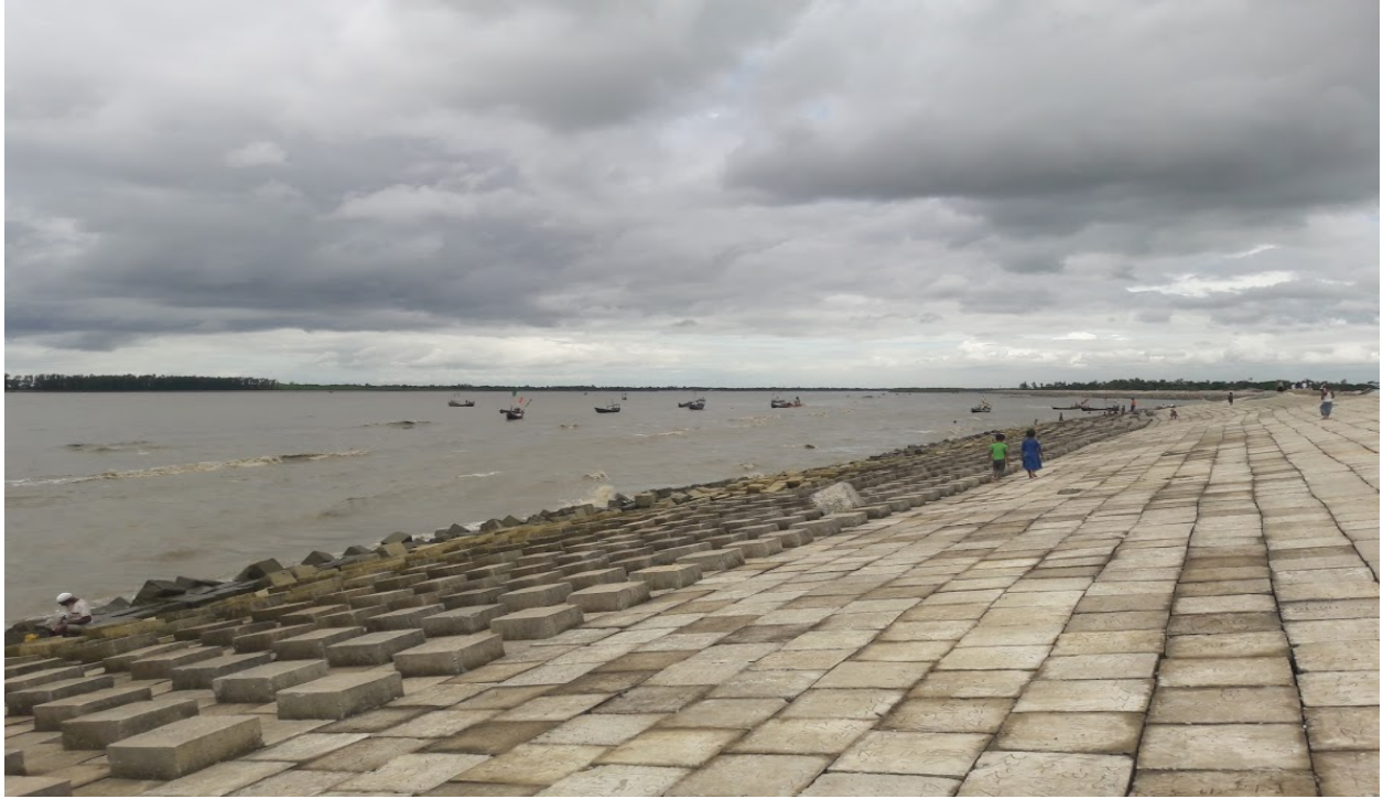
Figure: Bank Revetment process to reduce Erosion in the Study area
