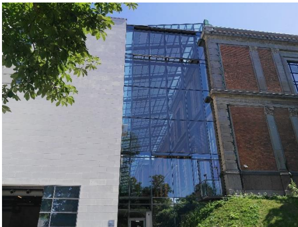
Figure 5: Connection between the old and the new part
