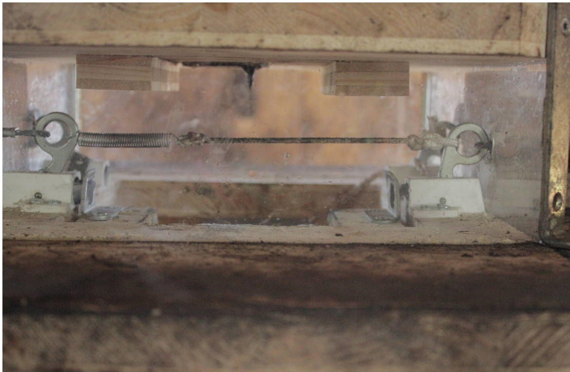
Figure 3: The opening mechanism consists of two metal latches on each side. Here the left one is in the "closed" position and the right one in the "open" position.
