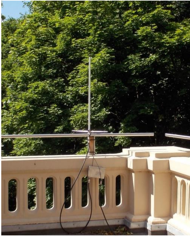
Figure 38: Omnidirectional antenna and dual band frontend amplifier mounted on the west side balcony of the IfA building
