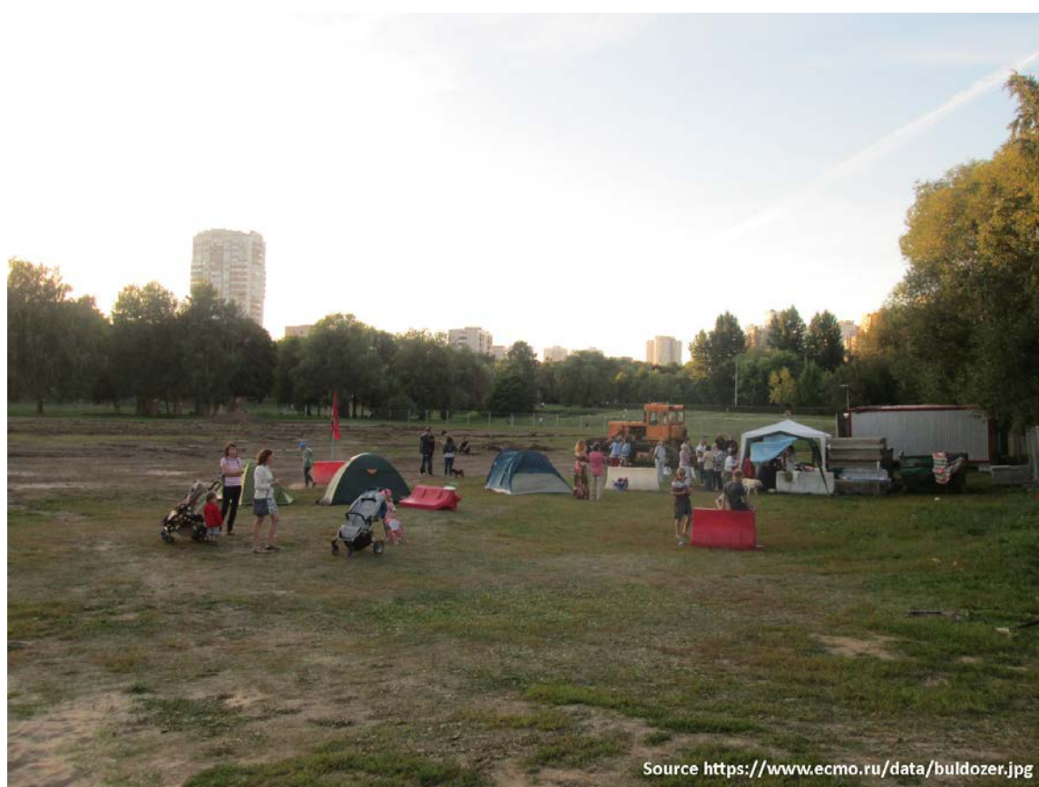
Figure 7. Activists are trying to occupy the construction site in Druzhba park
