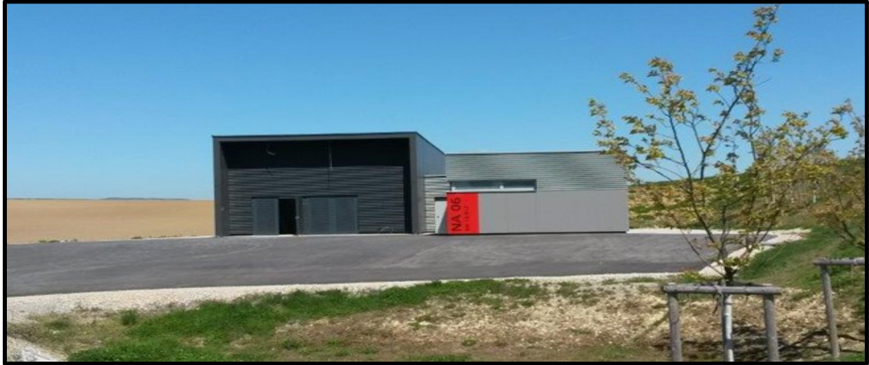
Fig. 23 Pummersdorfer tunnel emergency exit: picture by ÖBB Infrastructure
