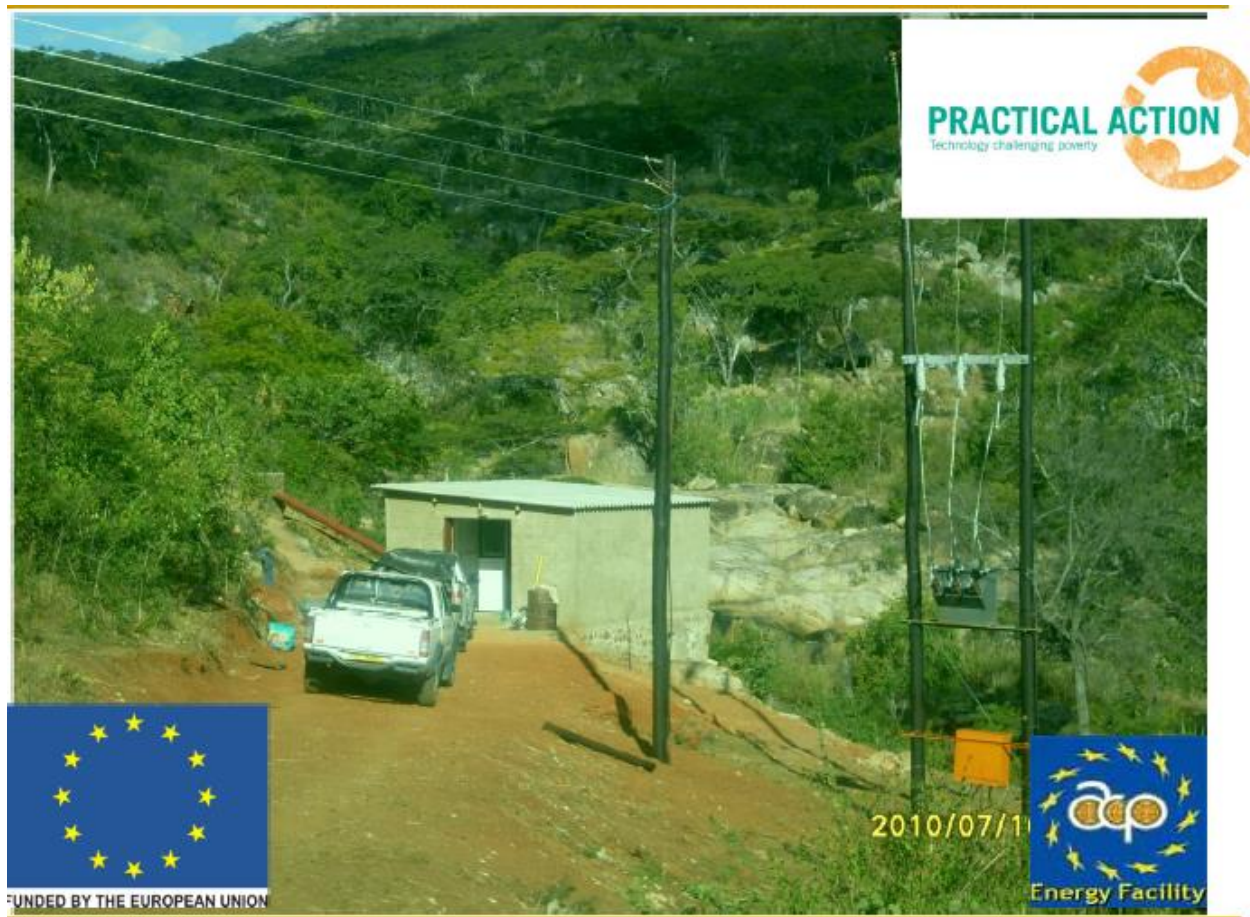
Figure 12: Turbine house, towards completion phase
