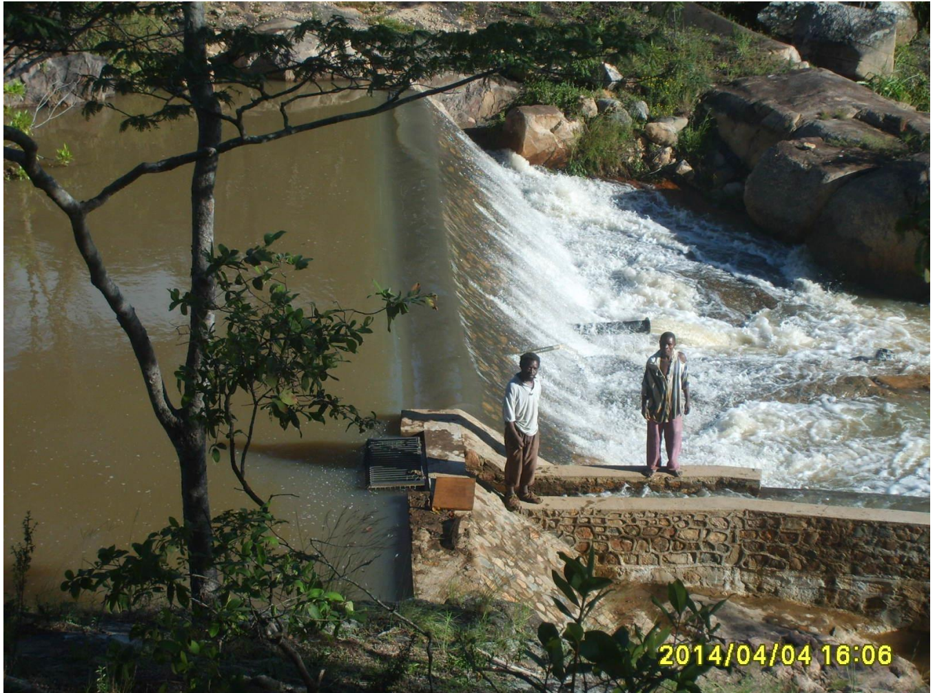
Figure 8: Mouth of the Penstock
