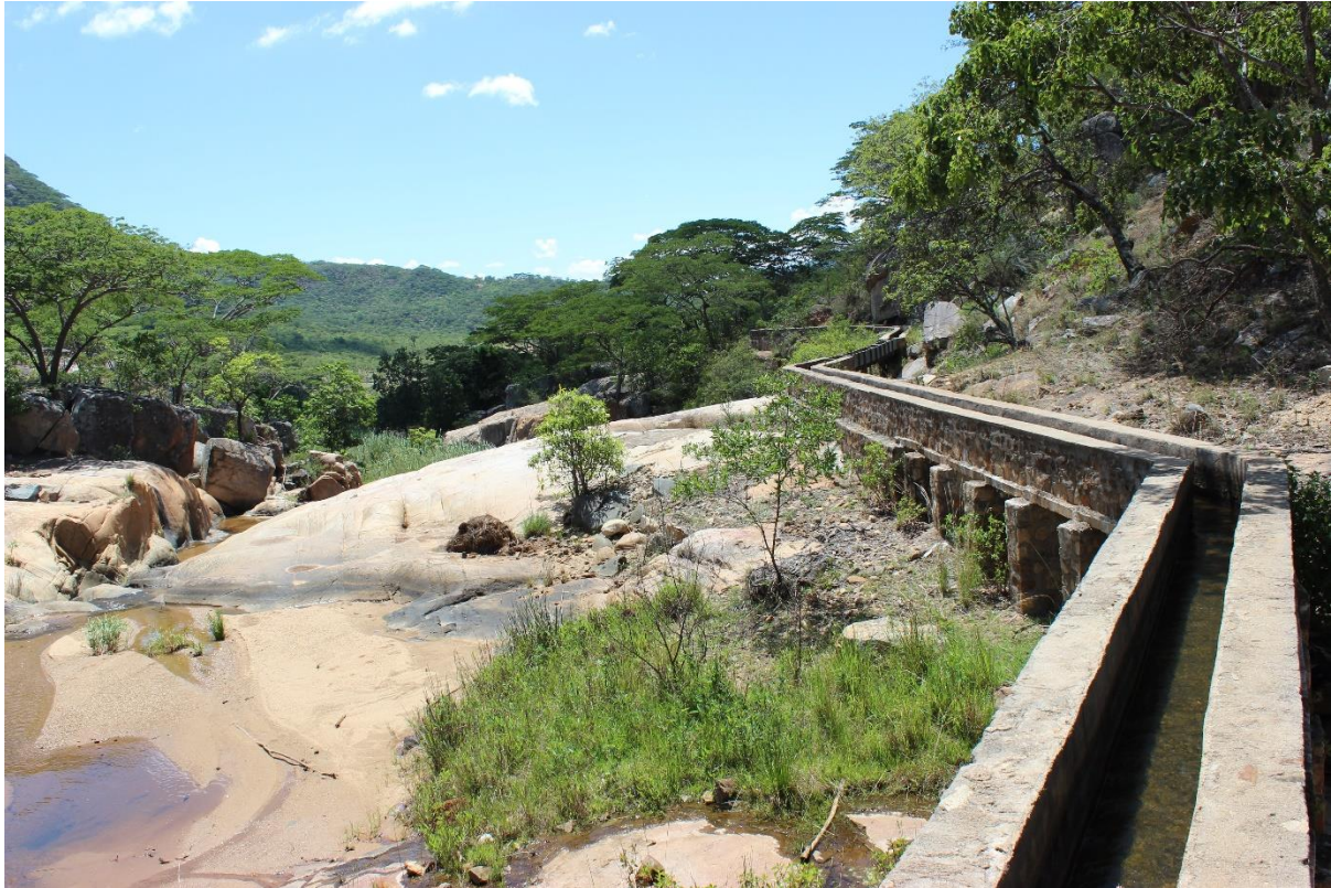
Figure 10: Civil construction work diverging water from the mouth of penstock
