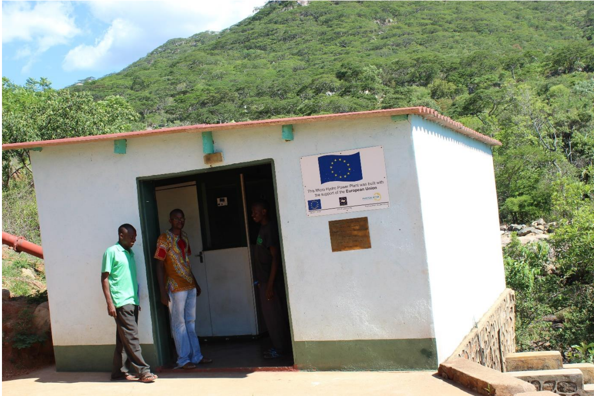
Figure 13: Turbine house after completion
