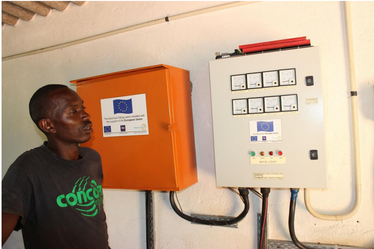
Figure 14: Power house worker observing meter readings
