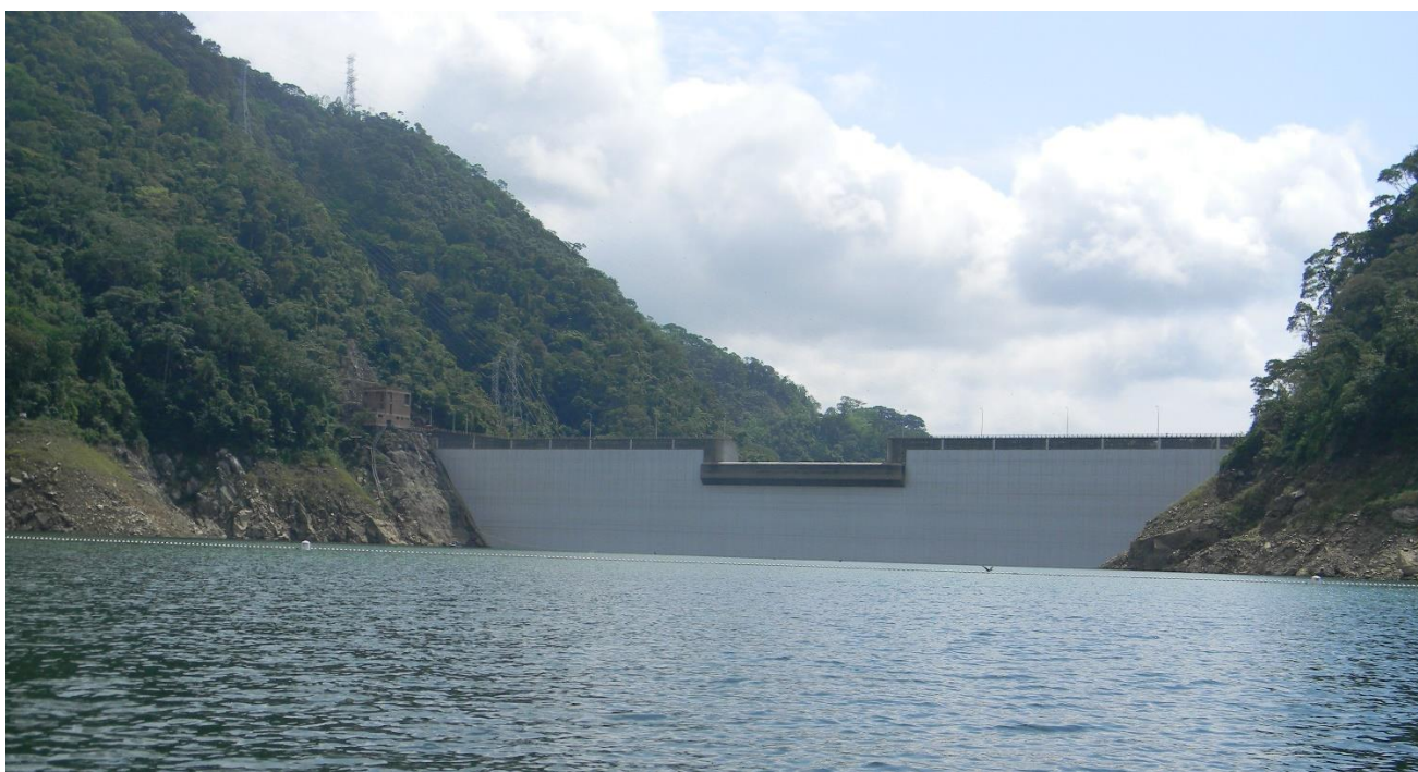
The Amani dam of La Miel I hydroelectric power plant
