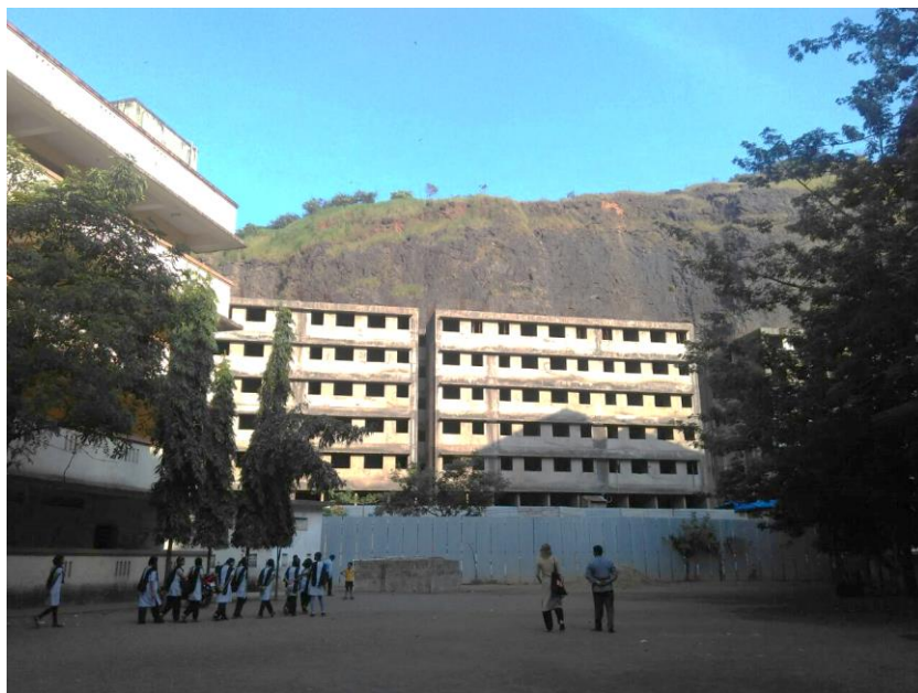
Figure 140: Front view of the new Buildings.
