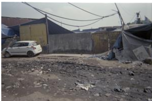
Figure 115: Illegally extended over ground water pipelines passing from roof to roof.
