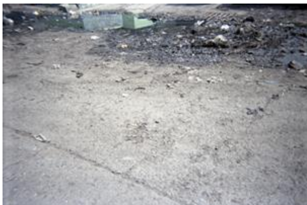
Figure 112: Dirty water puddles on the ground mixed up with waste.
