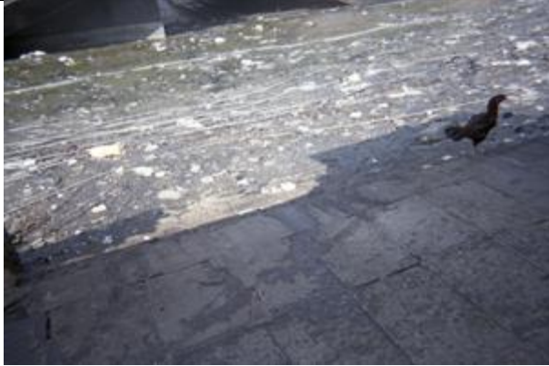
Figure 90: Illegally extended water pipelines at the creek.
