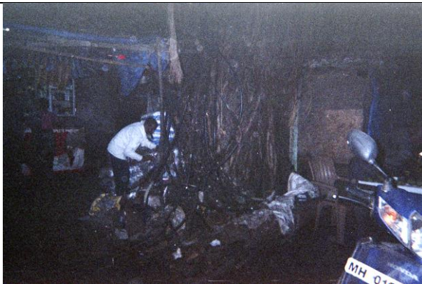
Figure 67: Bunch of water pipelines.
