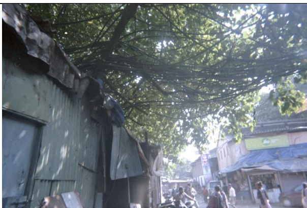
Figure 79: Illegally extended over ground water pipelines.
