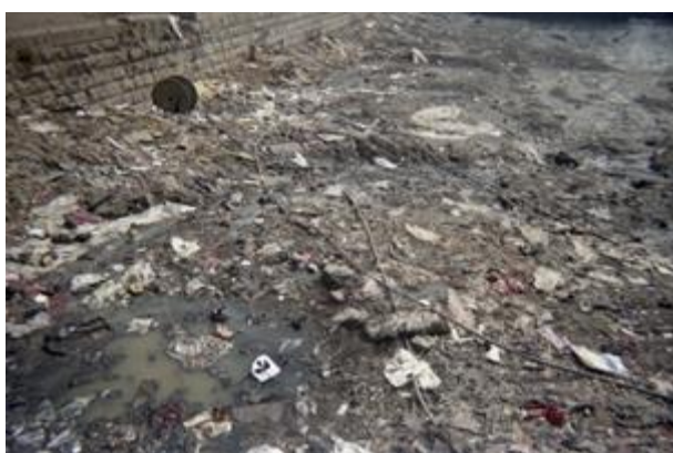
Figure 126: Pipelines passing a dumping site.
