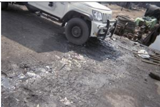
Figure 62: Water running to the surface from the burst of an underground water pipeline.
