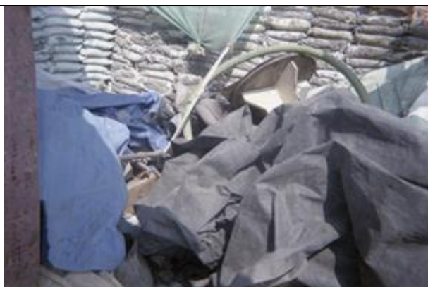
Figure 49: Hidden water pipeline.
