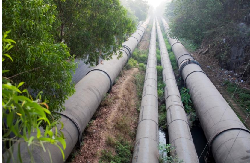
Figure 8: Water mains laid to transport water from the lakes to Mumbai. (Pani Haq Samiti, 2016b)
