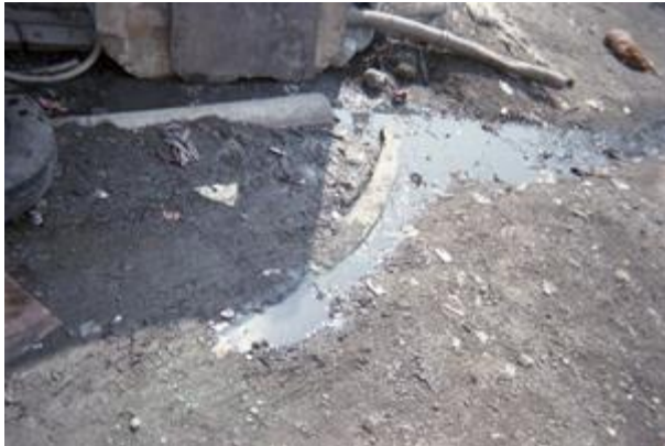
Figure 57: Sewage water on the ground.
