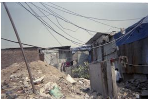
Figure 114: Illegally extended over ground water pipelines passing from roof to roof.
