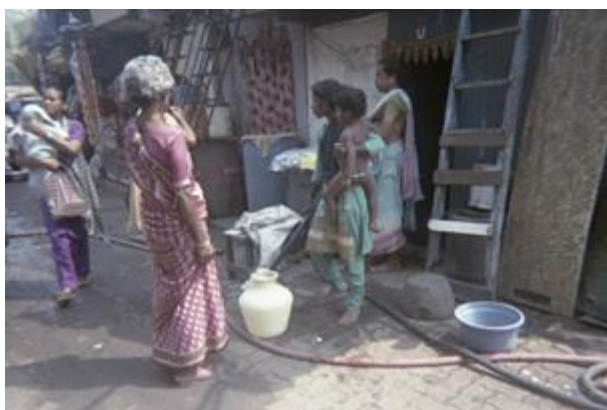
Figure 127: Water pipelines are laid to the doorstep through the vast connection of several pipelines.
