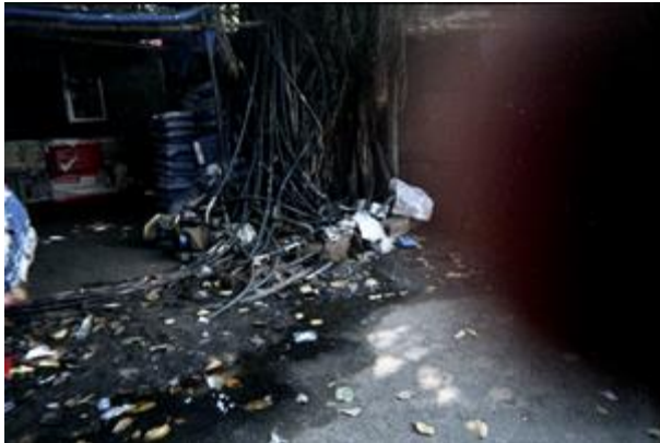
Figure 102: Bunch of water connections with motors hidden under the plastic bags.
