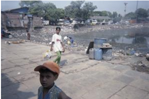
Figure 121: Water stored next to the dumping site and sewage disposal. Pipelines crossing the dumping site.
