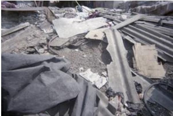
Figure 50: Hidden water pipelines
