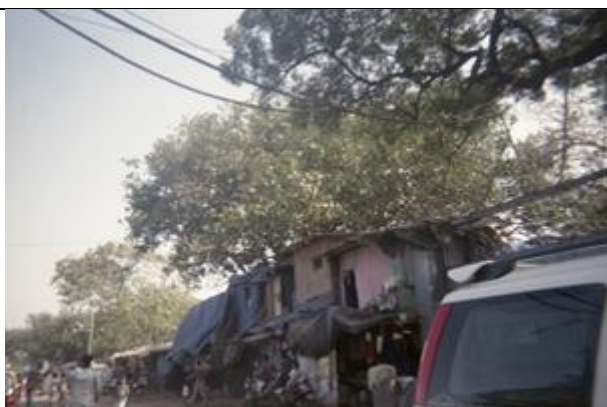
Figure 82: Illegally extended over ground water pipelines.
