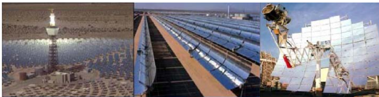
Figure 3. CSP Technologies (from left: solar tower, parabolic trough, and dish-stirling)
