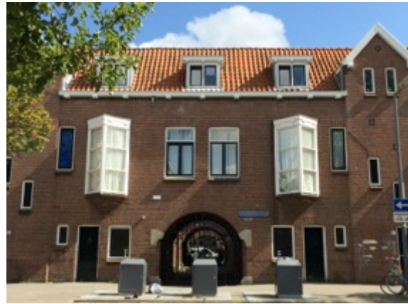
Figure 8 Outer ring of the Patrimoniumshof, own picture, 2014.
