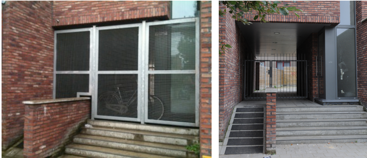
Figure 14 Fences: on the left the new situation, on the right the old situation. Source: own pictures, 2013 and 2014
