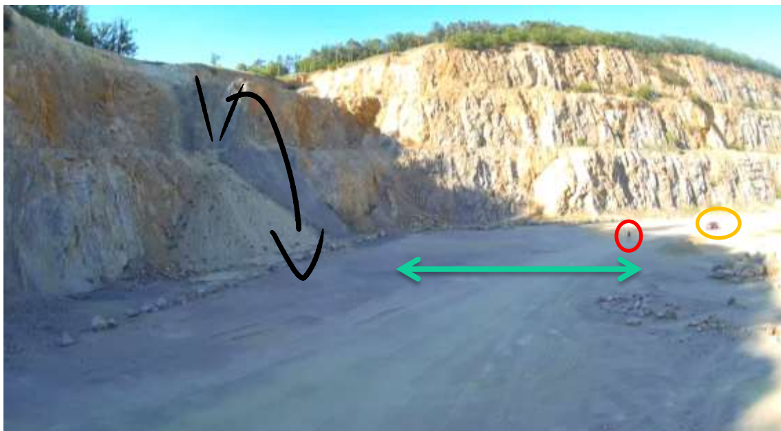
Figure 1: Working safety; potential rock fall (black), operator (red), car (orange), safe distance (green); note: picture taken from UAV
