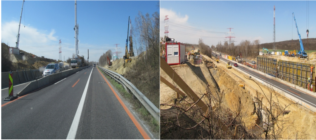
Fig. 3: Construction of the wildlife crossing
