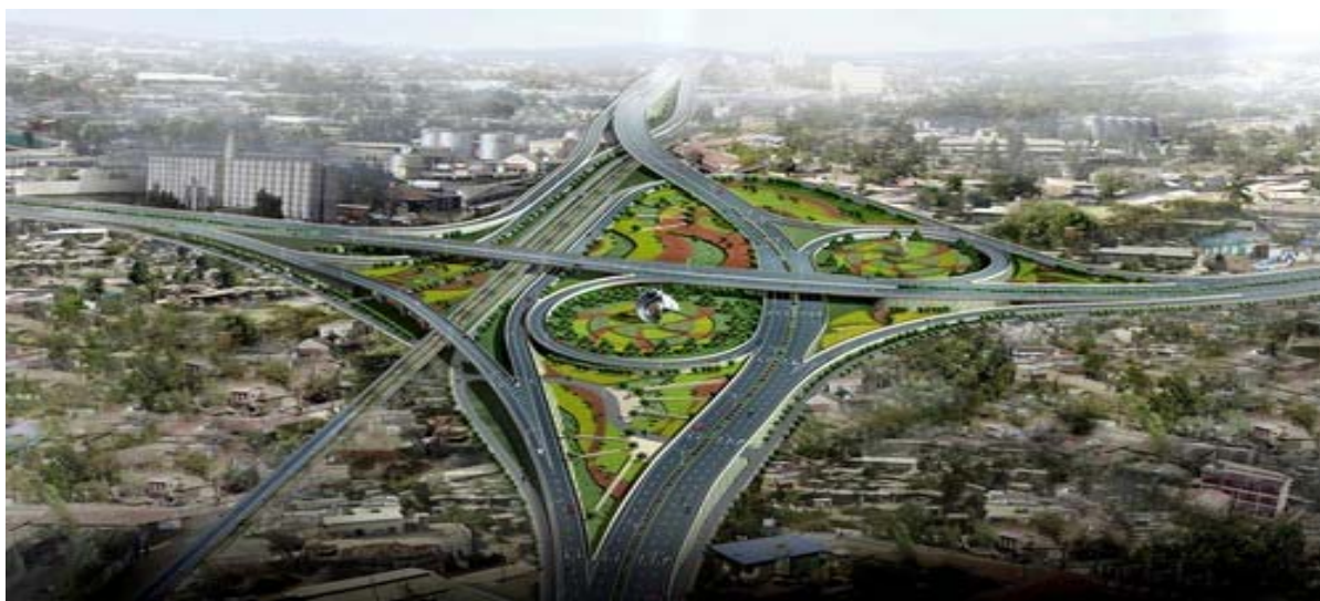
Figure-5: Gotera Interchange
