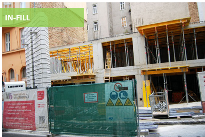
Fig. 20: In-fill Residential Development Advertised by Proximity to Naschmarkt in Mariahilf (own picture: 2013)
