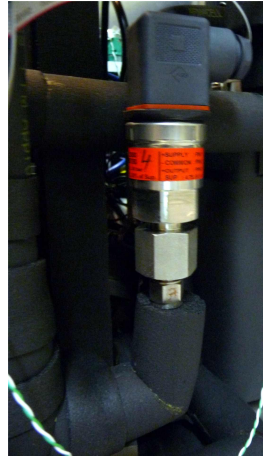
Figure 4.21: An assembled pressure transmitter AKS 2050 (Danfoss).
