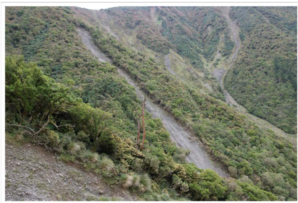
Figure 6.18: Landslide 2 situated in dry creek, seen from the opposite valley flank. It ranges from left upper corner to right lower corner.
