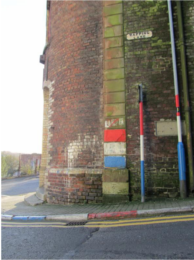
Fig. 23. Wapping Lane Entrance into the Fountain (my photo, 2011).
