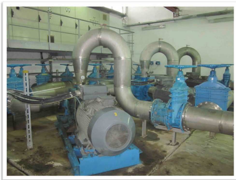
Picture 6: Pumping Station in the well-field, pushing water into the network and onto the Tepe hills.(Photo: C. Stubenberg)
