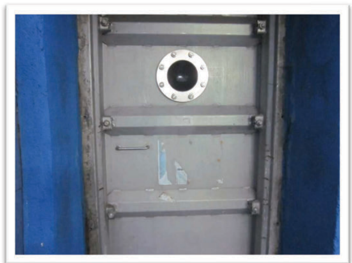
Picture 3: Bull-Eye window in steel pressure door. (Photo: C. Stubenberg)
