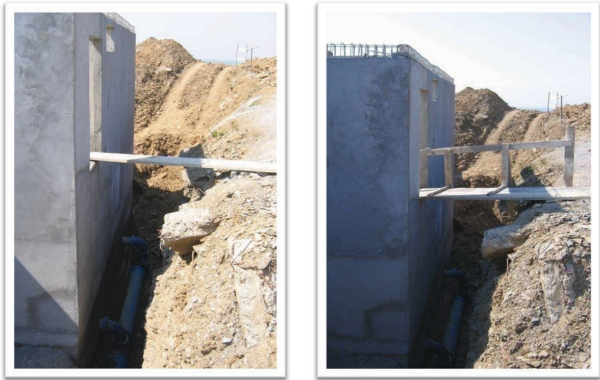
Picture 24: Wooden Bridge with and without safety measure. (Photo: ADA Project Archive)
