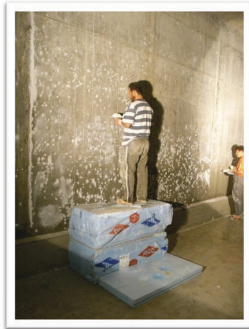
Picture 27: Workers closing pores with special cement inside the reservoir (Photo: ADA Project Archive)
