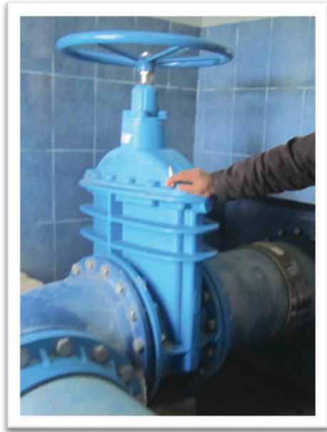
Picture 15: Hawle gate valve with an engineers hand. (Photo: C. Stubenberg)
