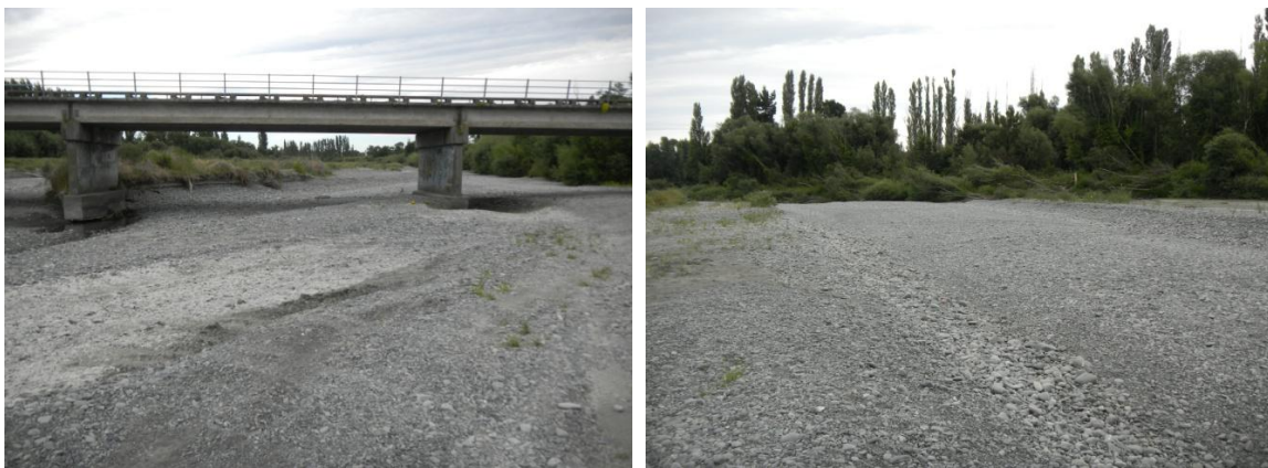
Figure 31 Dry riverbed at Digbys Bridge on January 5 th 2012 (left: upstream, right: downstream)
