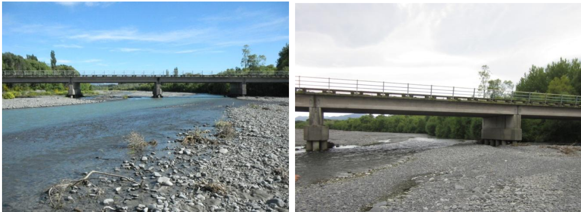
Figure 29 Flow at Thompsons Track Road (left: 25 th Nov 2011 and right: 5 th Jan 2012)
