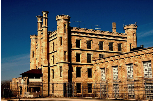
Abb. 6: Joliet Correctional Centre 133
