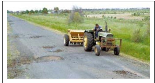
Fig.64, salt damage to roads, photo by author, both
