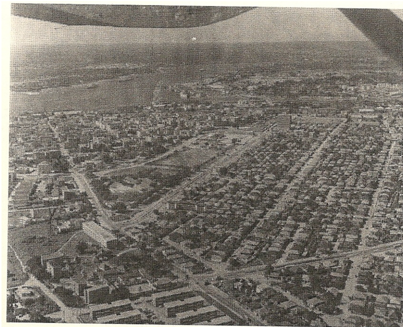
Figure 5.1 Aerial view of Kariakoo/City Centre/Harbour circa Independence
